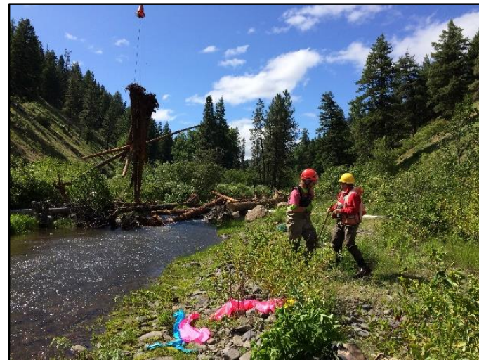
Helicopter placing large wood jam structures
