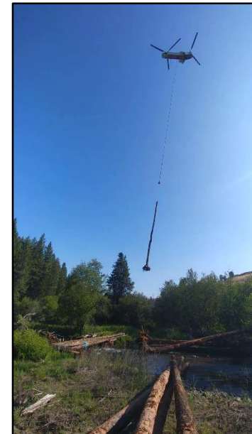
Helicopter placing large wood jam structures
